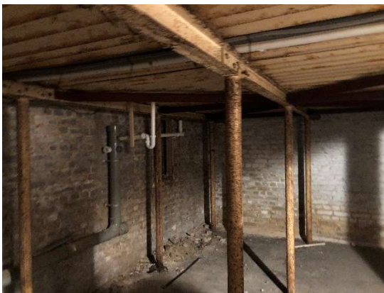
Photos 16 & 17: Basement areas needing improvement to house ventilation plant
