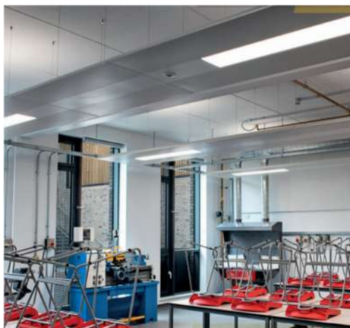
F Figure 7: Multi-service suspended raft in use
