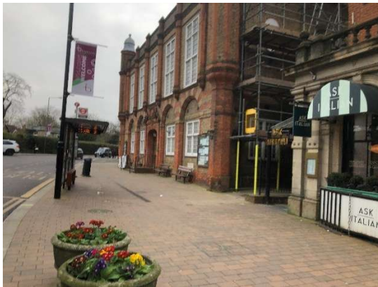
Photo 1: Main Street Approach
