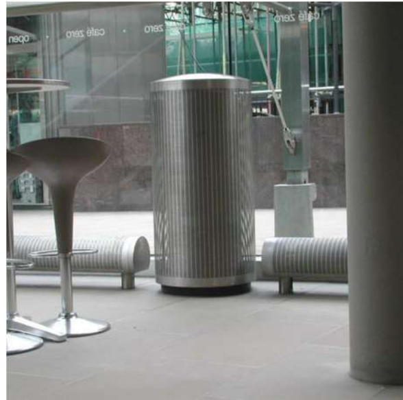
Figure 2: Range of displacement vent terminals Figure 3: Typical freestanding vent terminal
